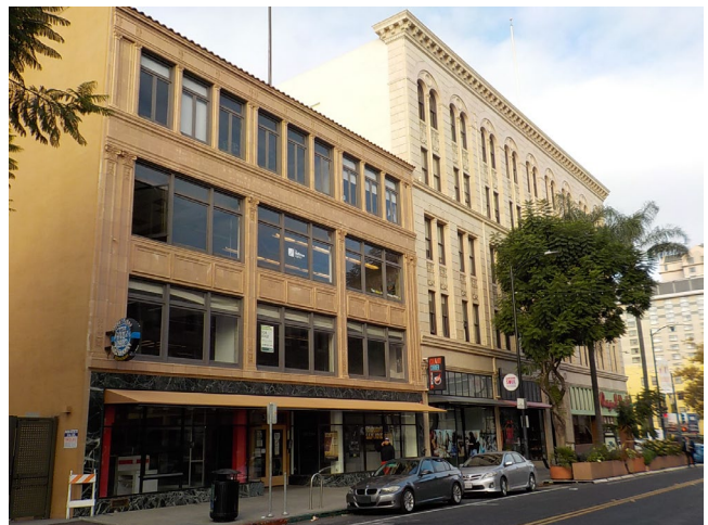
30. Commercial Building Adjoining South (to left) and Commercial/Residential Building Adjoining East (to right)
