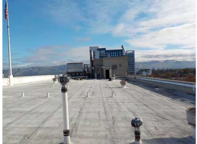
8. Building Roof (6-Story Portion of Building)
