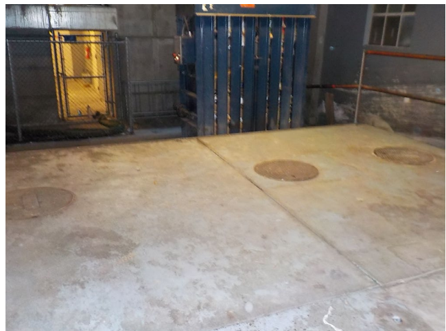
6. Eastern Loading Dock with Grease Interceptor in Dock and Box Crusher Adjoining Dock
