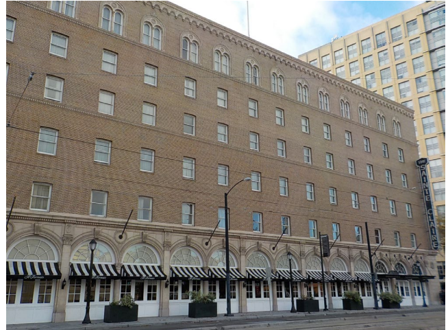
2. Northern Façade of Building
