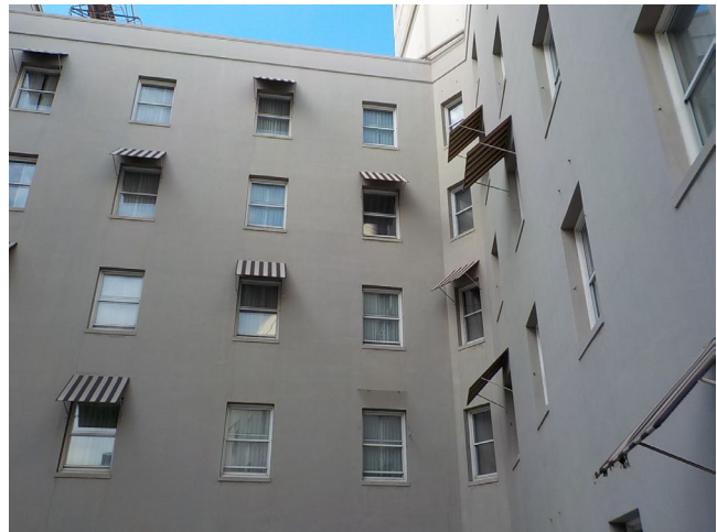
4. Southern and Eastern "Interior" Façades of Building
