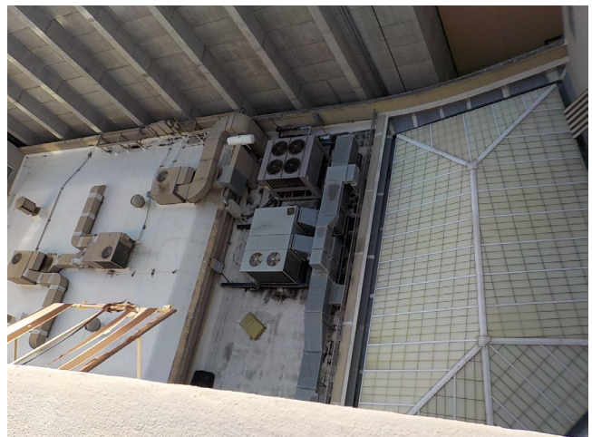
12. Building Roof (Single-Story Portion of Building)
