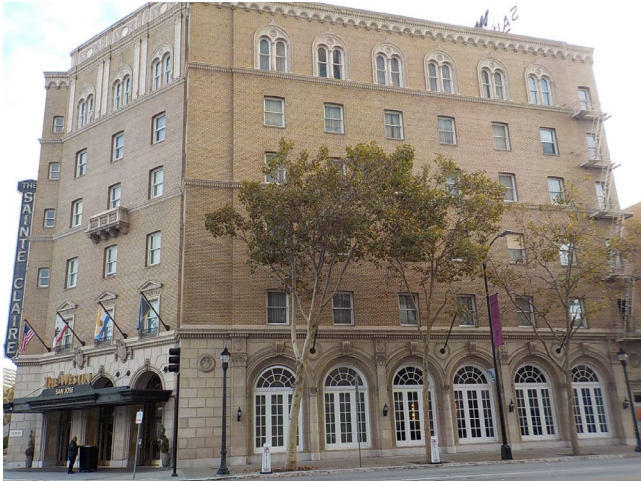
1. Northwestern and Western Façades of Building
