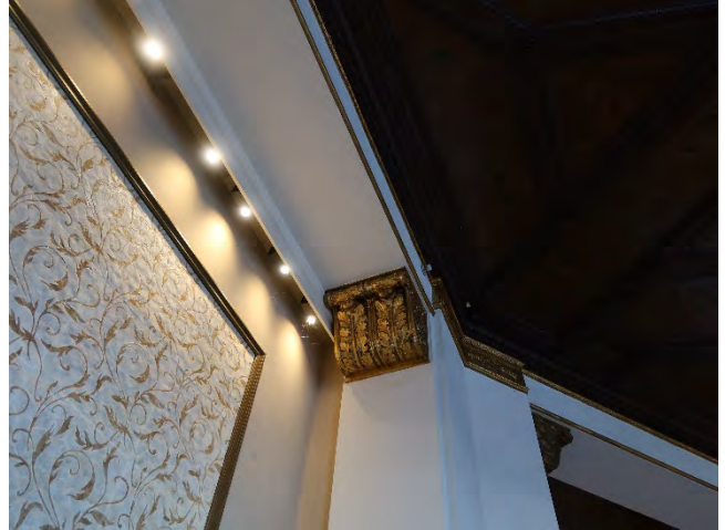
32. Painted concrete columns and beams with decorated bracket.
