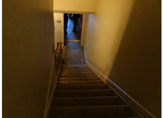
38. The central stair.
