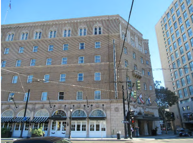
1. The west part of the north elevation. Main entrance is in view on the northwest building corner.
