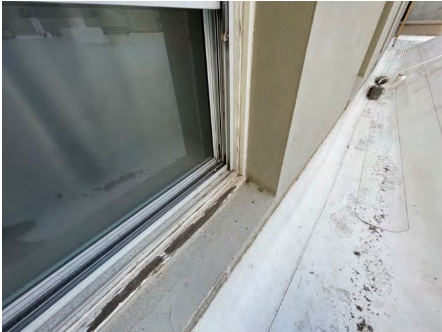
E - 36: Aluminum window at the back side
