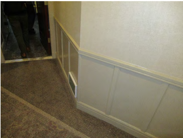
33. Typical finishes in upper floor corridor, second through sixth floors.
