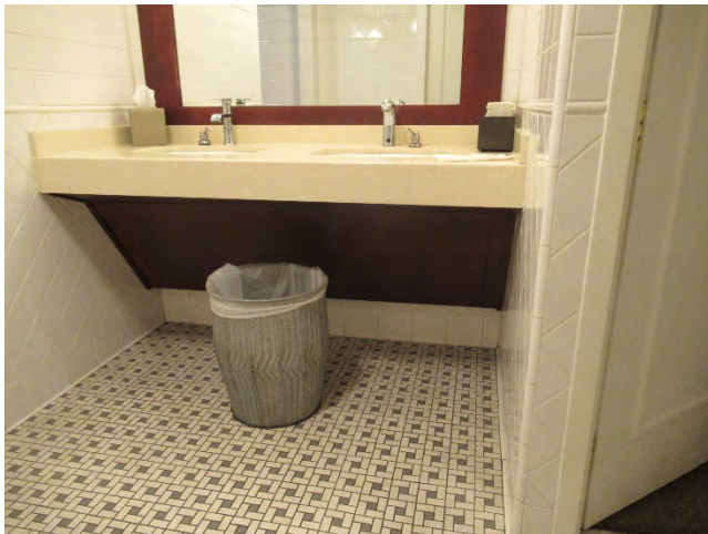
105. Protected knee clearance is provided at restroom lavatories.
