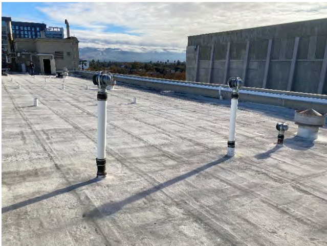
M-9. Corridor ventilation fans.
