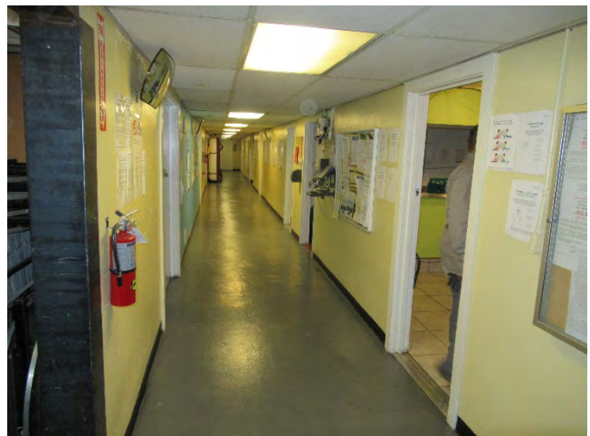
78. The basement corridor in the back-house section.
