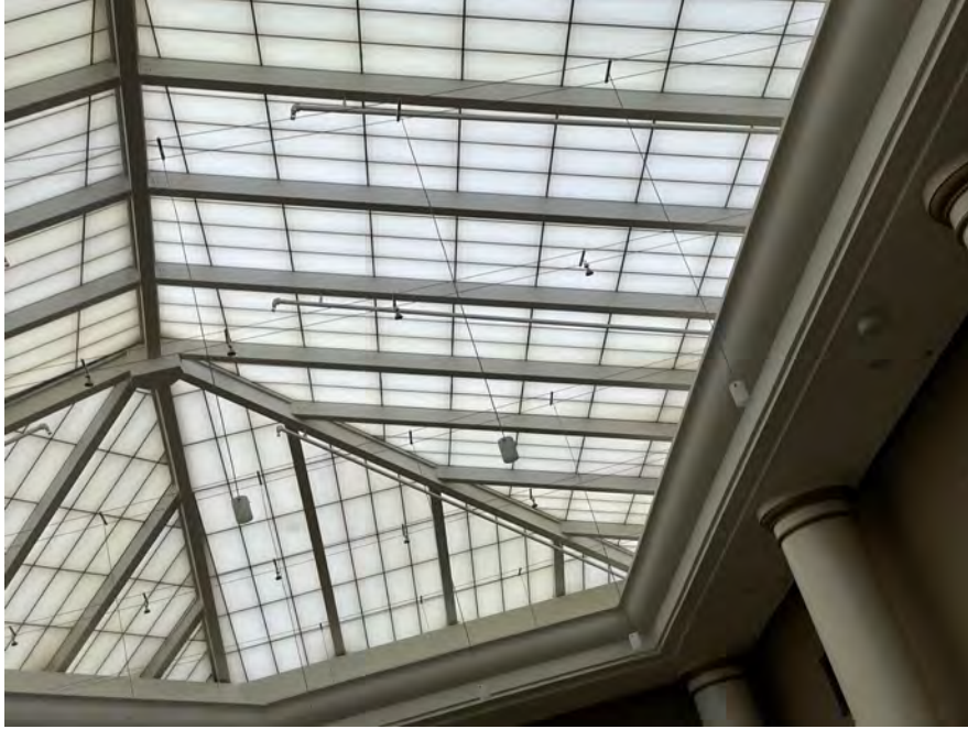
E - 15: Underside of Skylight
