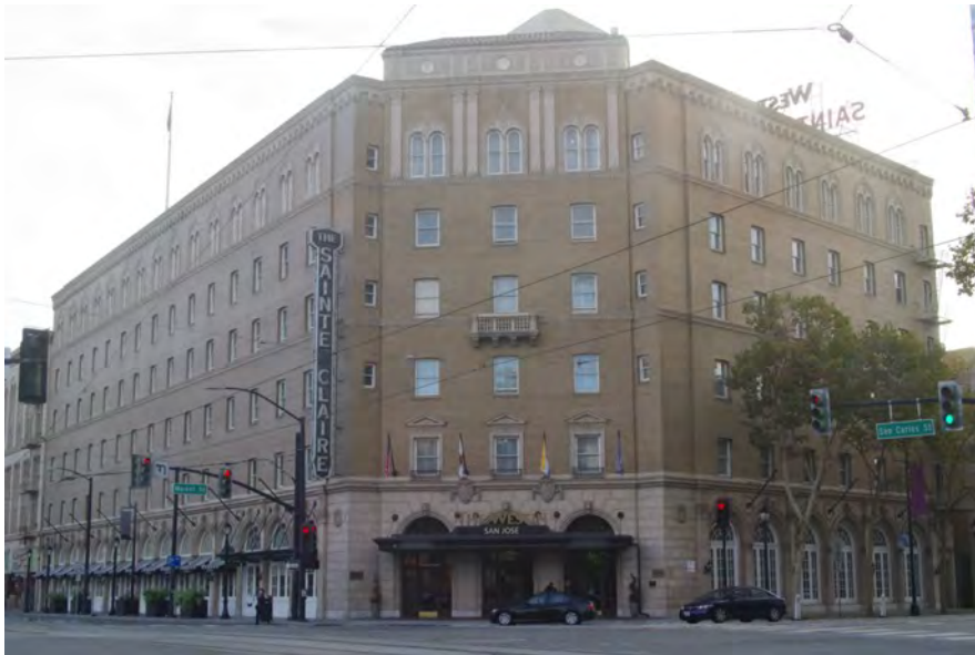
E - 22: Street Façades
