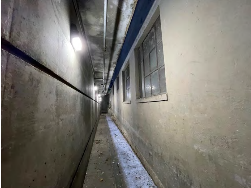
E - 25: Painted concrete at back wall
