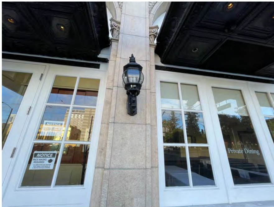
E - 38: Doors at the storefronts
