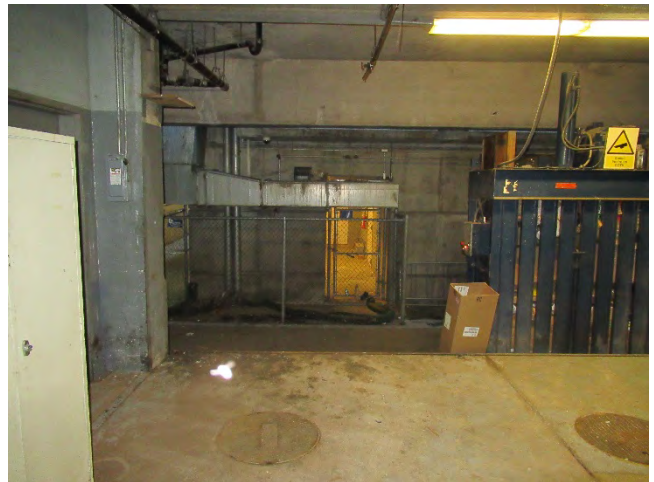
94. The Loading Dock near the basement southeast corner.
