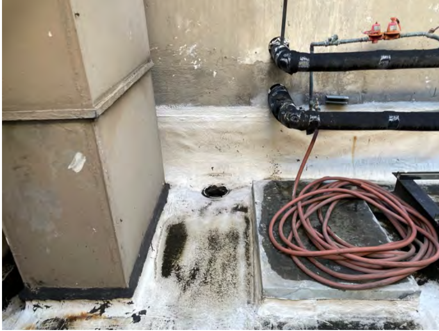
E - 11: Coating over top of base flashing
