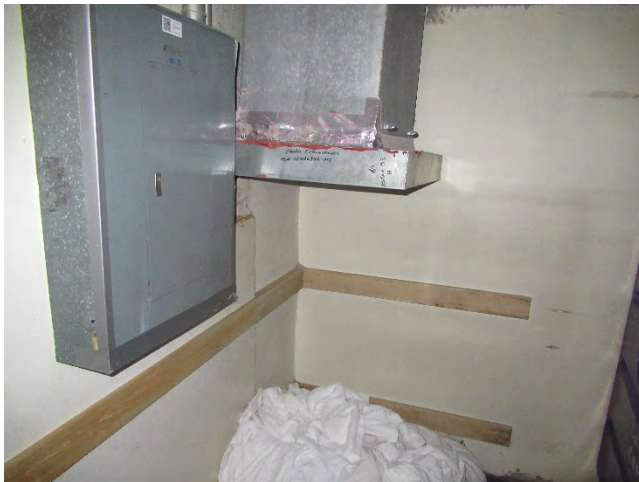
93. The laundry chute bottom near the Basement Laundry area.
