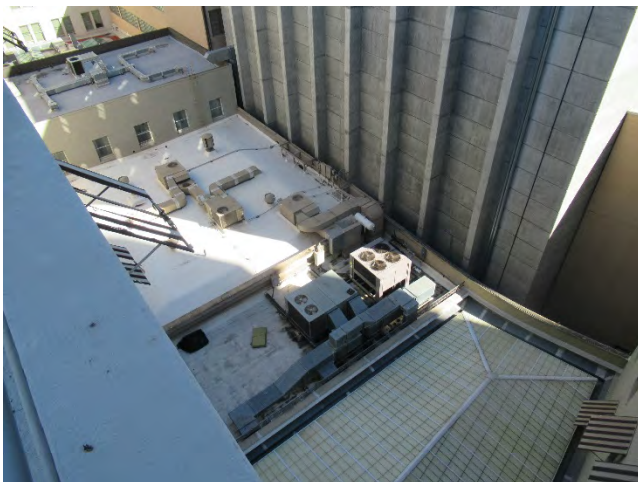
17. The lower roofs seen from the main roof. From left: the Sainte Claire Ballroom is the only second floor space; the Grand Ballroom A & B roofs; the Atrium roof is one large skylight.
