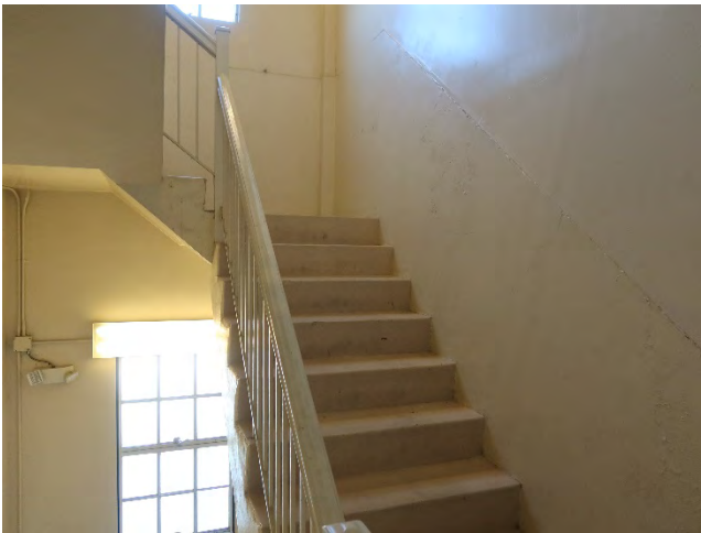
39. Typical finishes at utility or egress stair.
