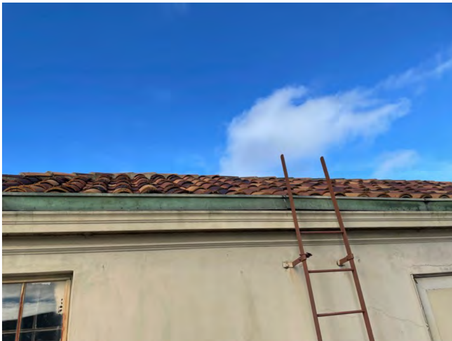
E - 8: Tiles at Penthouse storage
