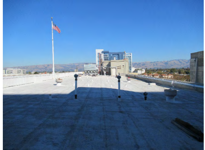
14. Looking east along the eastern leg of the roof.
