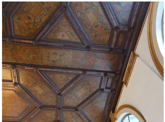
30. Decorated ceiling in the lobby.
