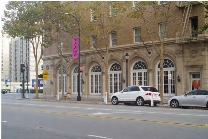
E - 34: Ground level windows
