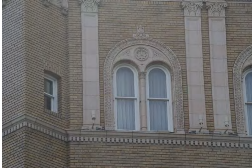
E - 33: Windows at Sixth Floor
