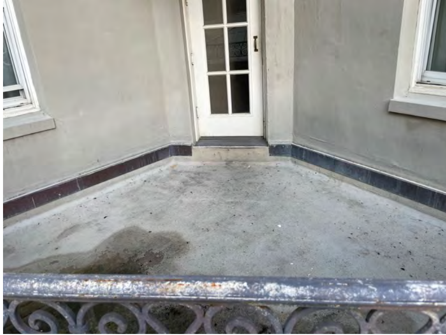
E - 17: Pedestrian traffic coating at small deck
