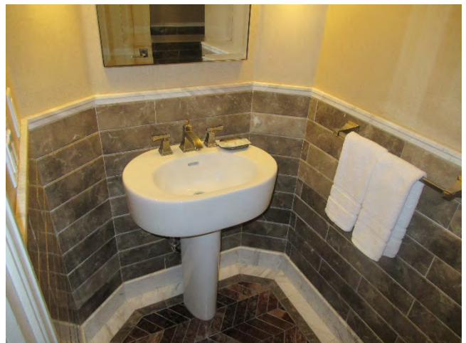
60. Finishes and fixtures in the Grand Suite bathroom.
