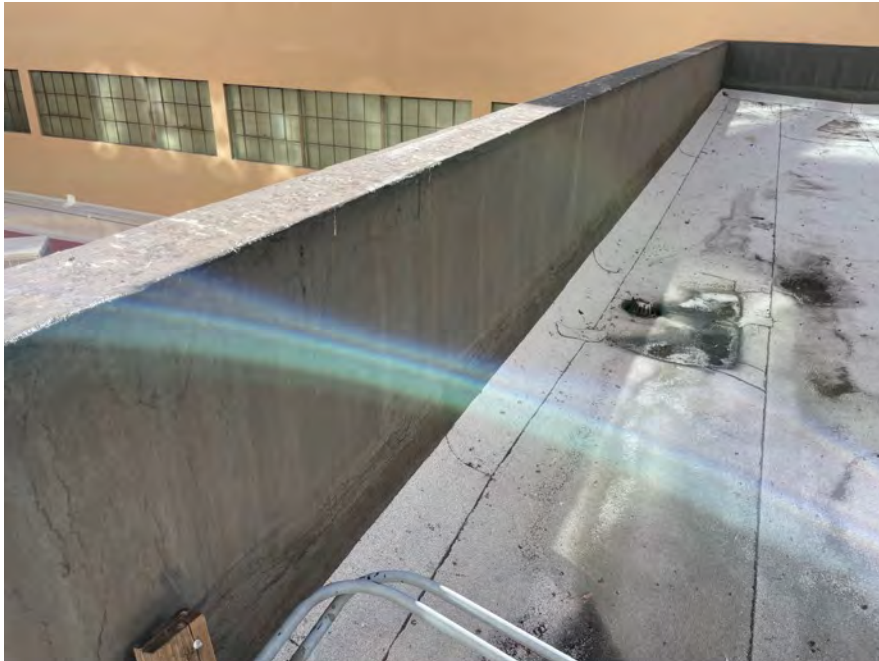
E - 20: Coating at parapet over base flashing
