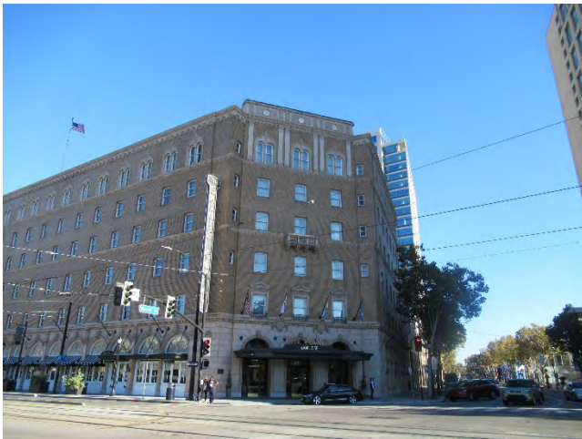
3. View of the northwest building corner from the northwest. Penthouse with sloped mission tile roof is in view at the top of the northwest corner.
