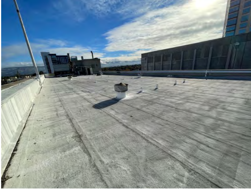
E - 1: Main Roof
