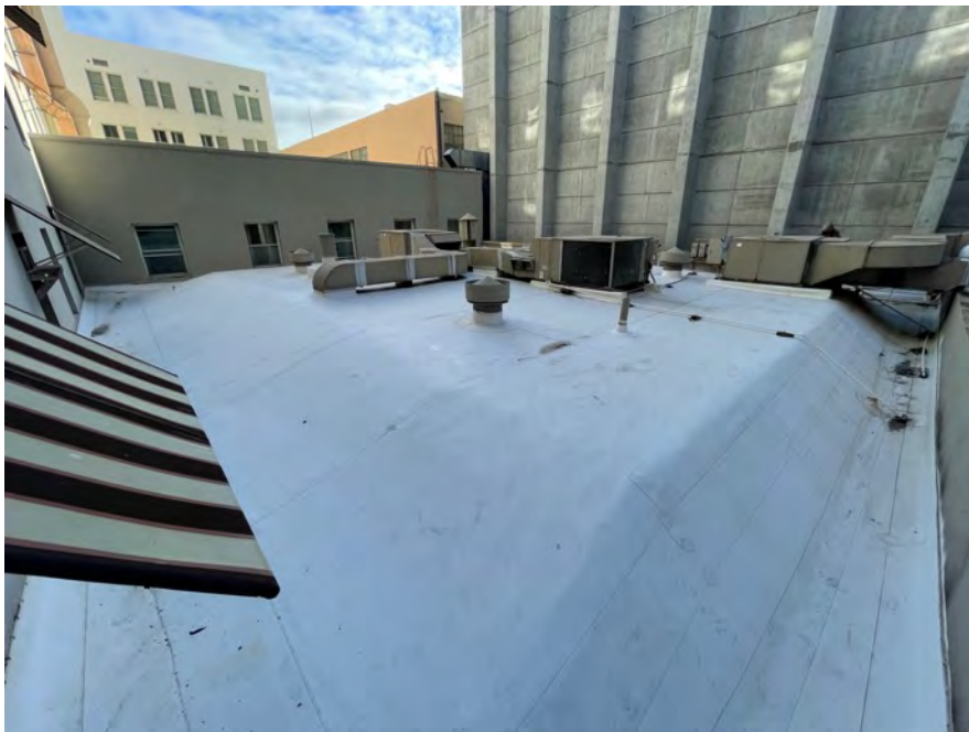
E - 12: Ballroom East Roof - TPO
