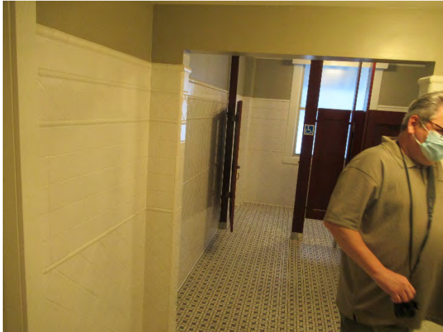
103. Accessibility in public restrooms is generally good.
