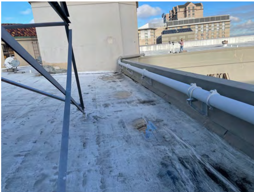
E - 4: Sloping at Main Roof
