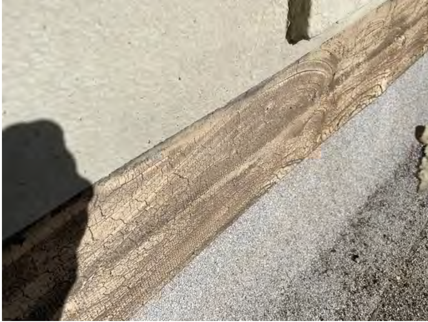
E - 19: Coating over base flashing
