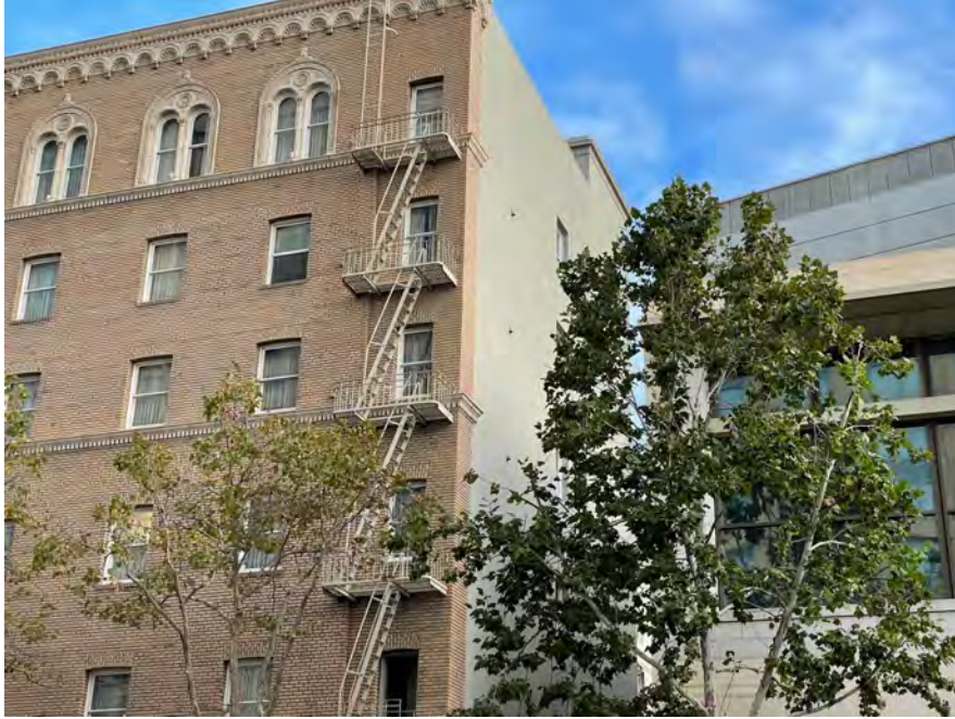
E - 23: Cement Plaster (stucco) at South Wall
