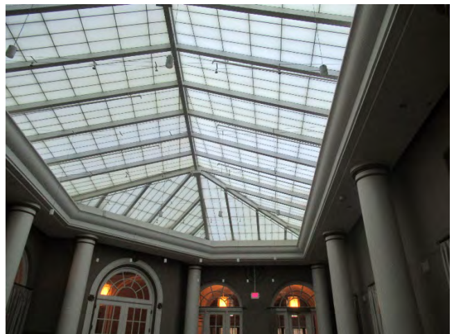
72. Most of the Atrium ceiling is a skylight.
