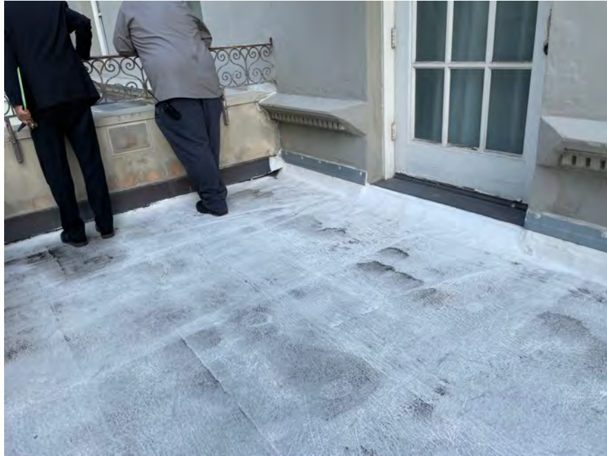
E - 9: Ballroom West Roof – SBS BUR
