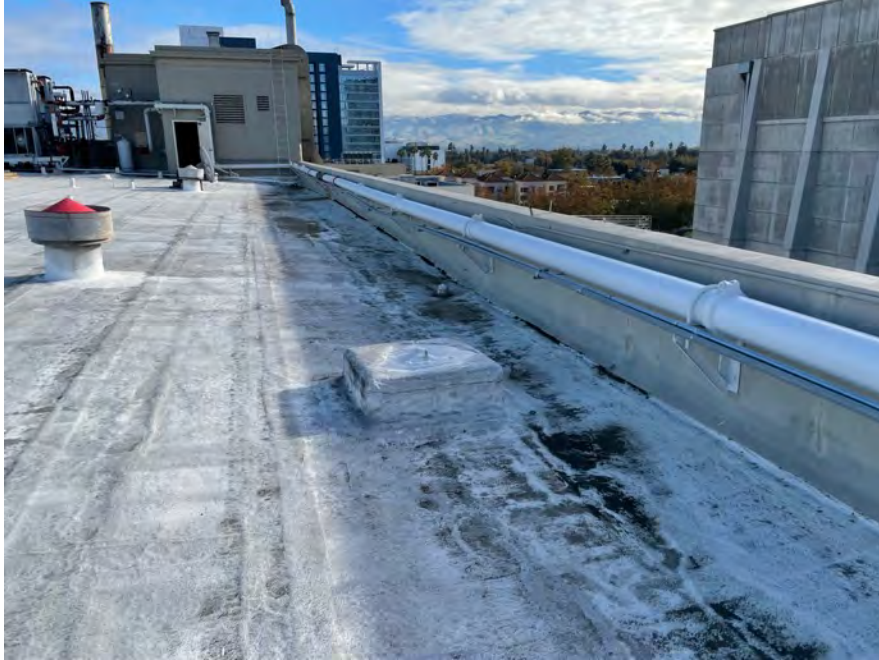
E - 3: Sloping at Main Roof
