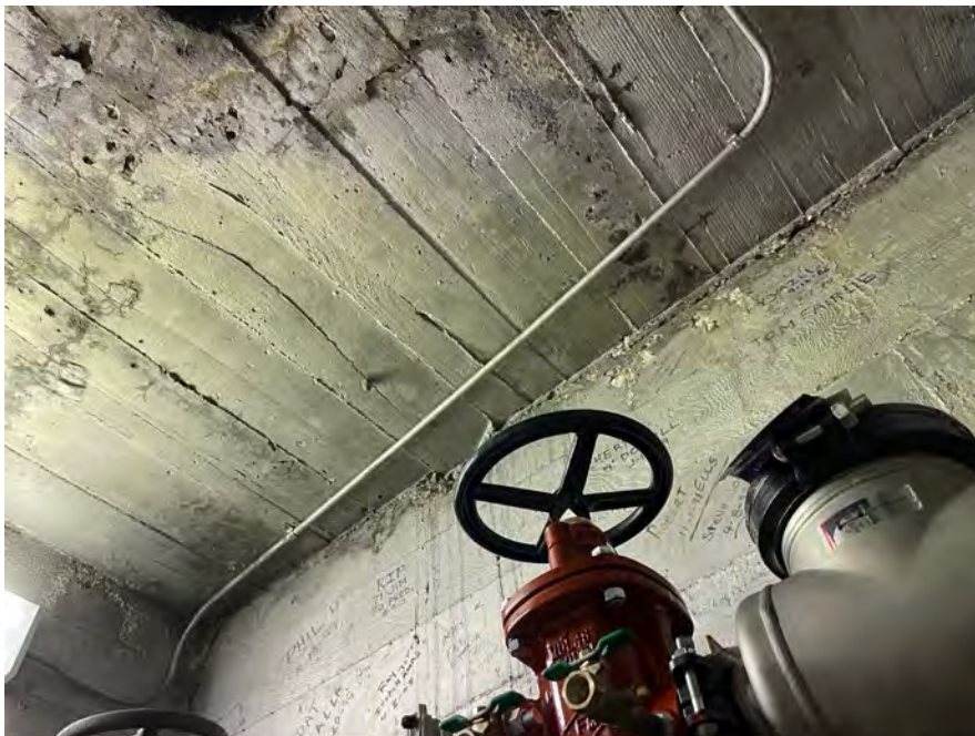
E - 40: Underside of sidewalk
