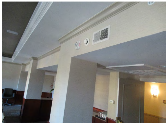
66. Columns and finishes in the Santa Cruz room. The center of the ceiling is a single raised coffer with concealed lights. Fire alarm horn and strobe in view.
