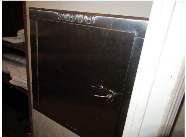
92. A laundry chute door in an upper floor Housekeeping Storage Room.
