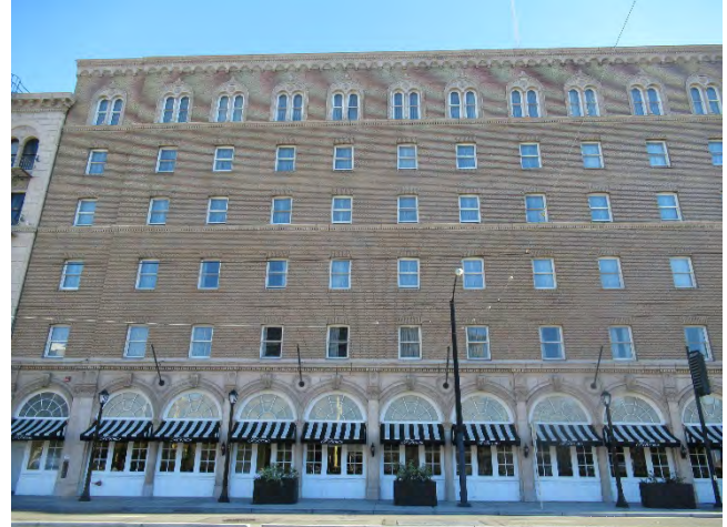
2. The eastern part of the north elevation.
