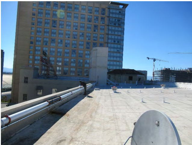
15. Looking west along the east leg of the roof.
