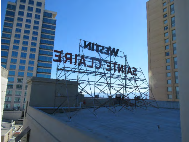
13. Looking south along the southern leg of the main roof.
