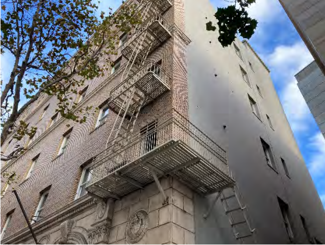
M-25. Exterior fire escape.
