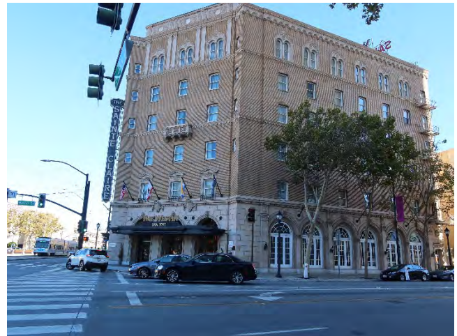
4. View of the northwest building corner and the west elevation.
