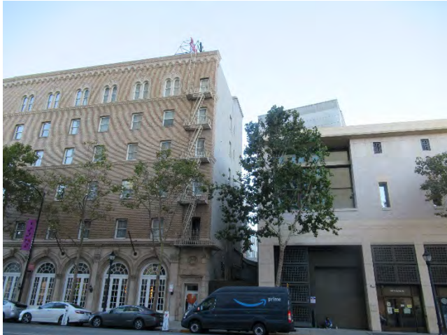
7. The south end of the west elevation. Part of the south elevation is in view. The building fire escape is in view.
