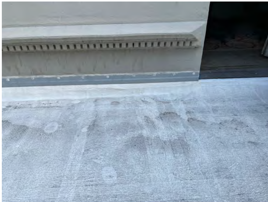
E - 10: Coating at base of wall
