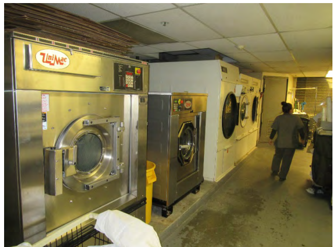
90. The Laundry Room in the basement.
